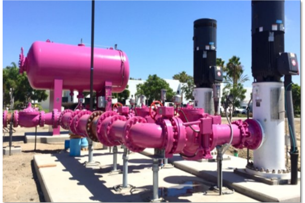
Closed surge vessel at a reused water pump station
