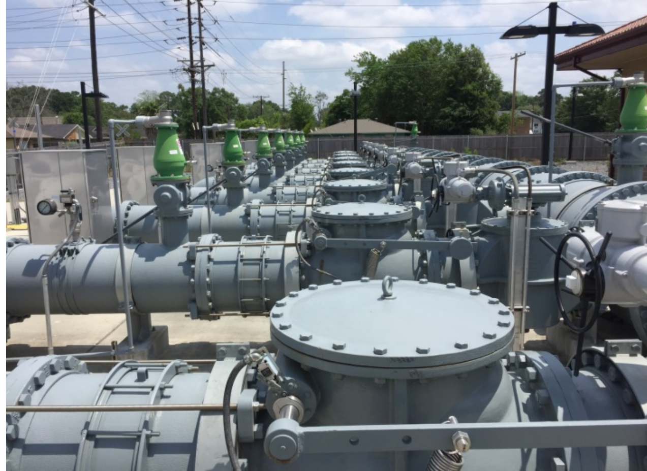
Vacuum breaker valves (in green, at left) at pump discharges
