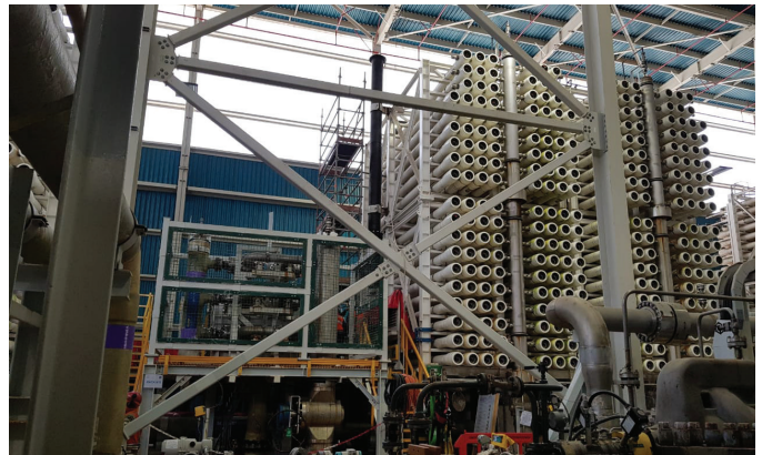
Figure 1: Image of one of the nine Reverse Osmosis (RO) racks as the chimney was being installed.
