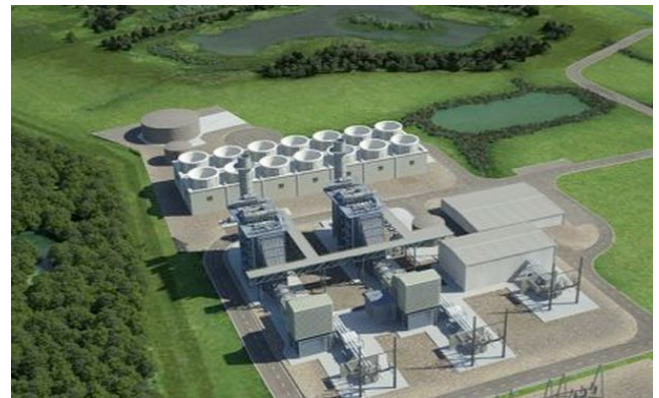
Woodbridge Energy Center, Woodbridge, NJ, USA
