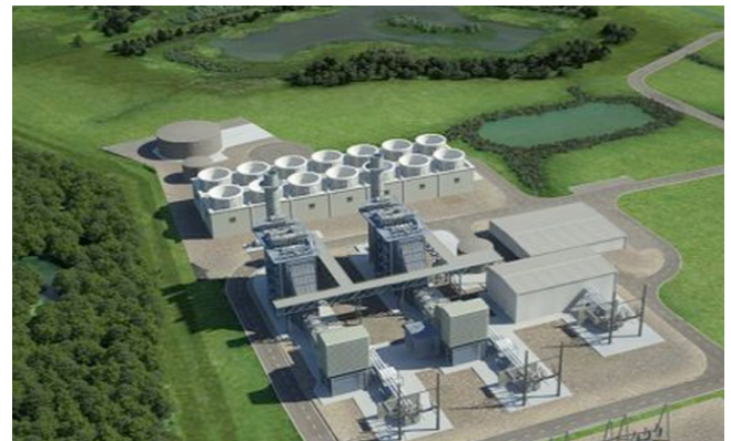
Woodbridge Energy Center, Woodbridge, NJ, USA
