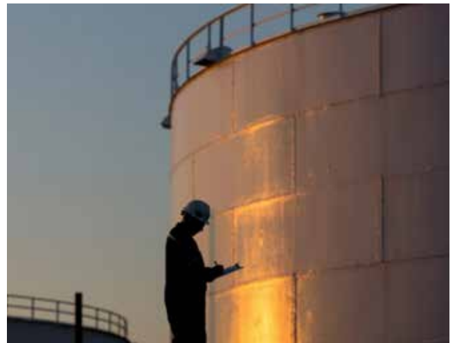
BP Tank Inspection - New Jersey
