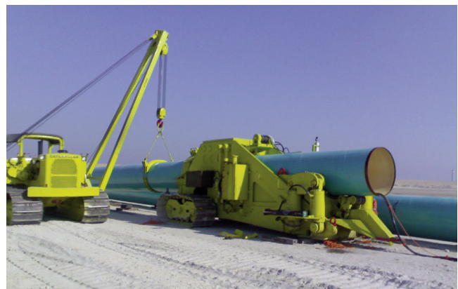
Figure 12. Pipeline Bending Process.
